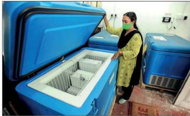
BBMP has identified Dasappa Hospital near Town Hall to refrigerate and store Covid-19 vaccines as and when they are shipped to the city. Vaccines will be stored here before they are dispatched to the government health centres. — N Narasimha Murthy
